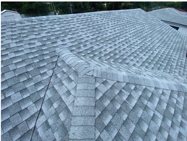
Asphalt shingle roof covering
