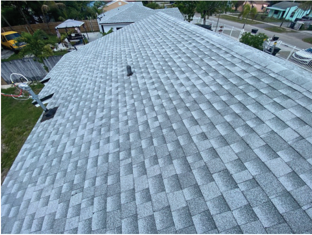
Asphalt shingle roof covering
