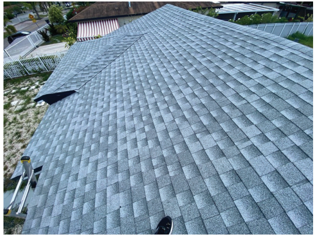
Asphalt shingle roof covering
