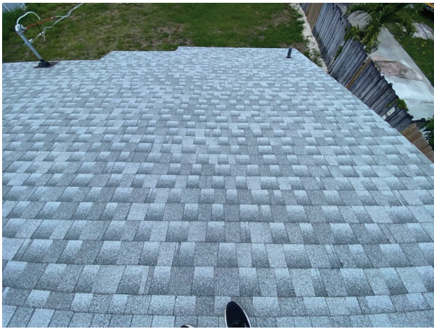
Asphalt shingle roof covering
