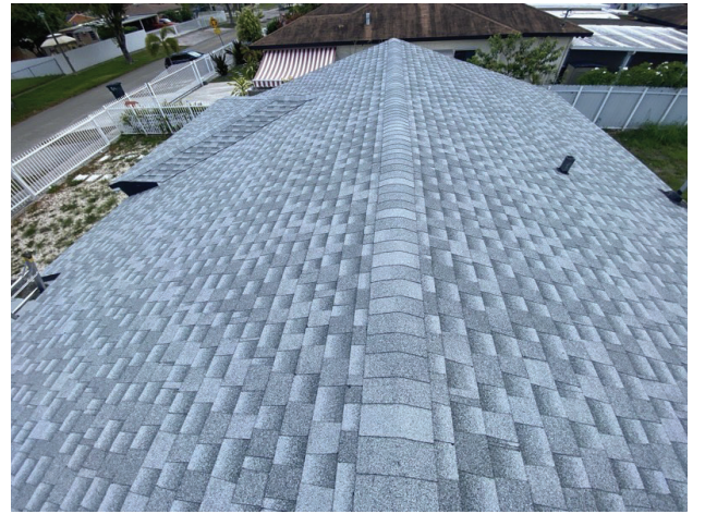
Asphalt shingle roof covering
