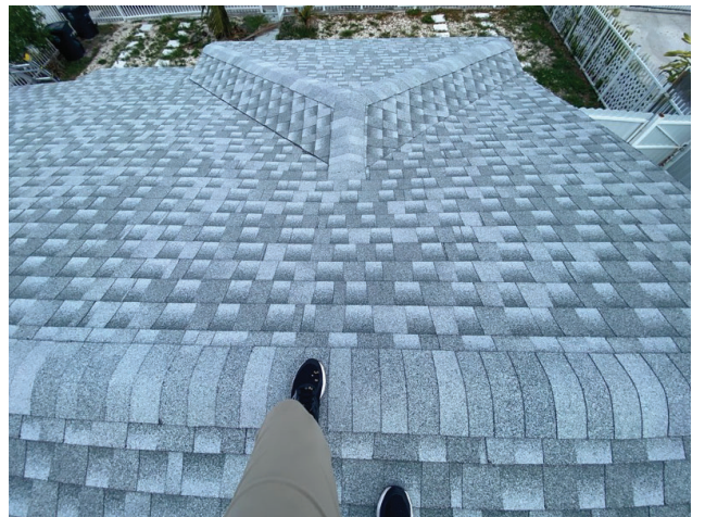
Asphalt shingle roof covering
