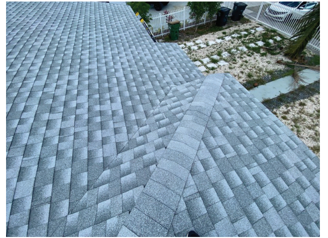
Asphalt shingle roof covering
