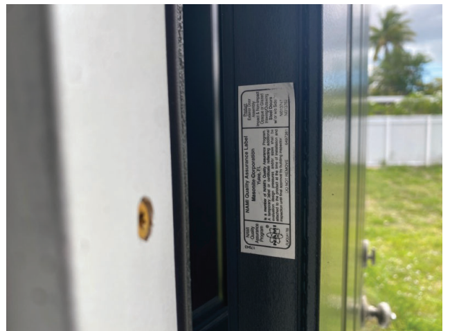
Rating label for rear solid impact opening
