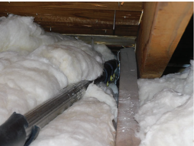
Roof to wall attachment (Single strap)
