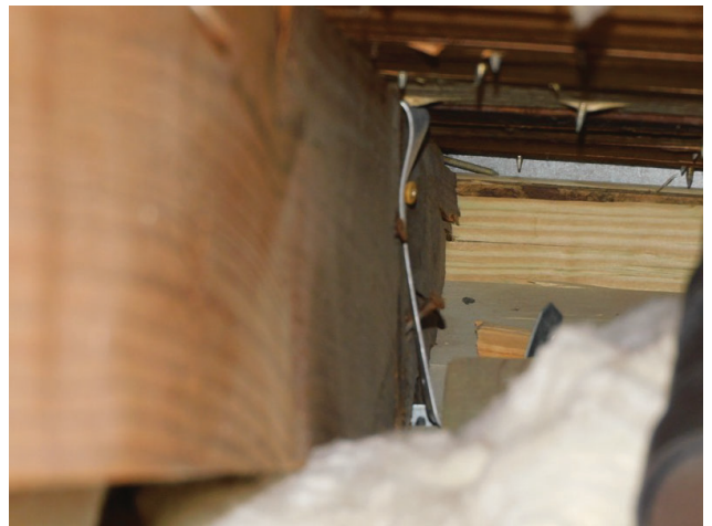
Roof to wall attachment (Single strap)
