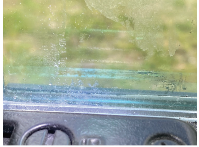
Rated etching for all impact glazed openings
