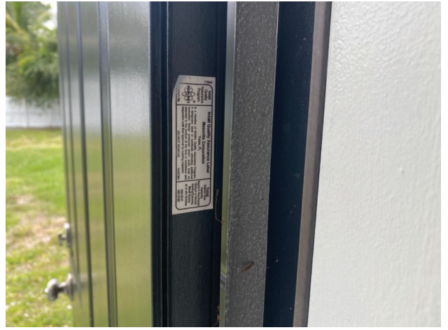
Rating label for rear solid impact opening
