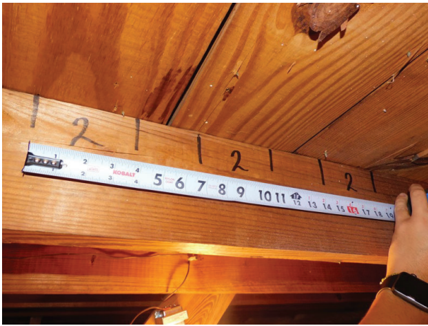
Roof deck attachment (Two nail per board)
